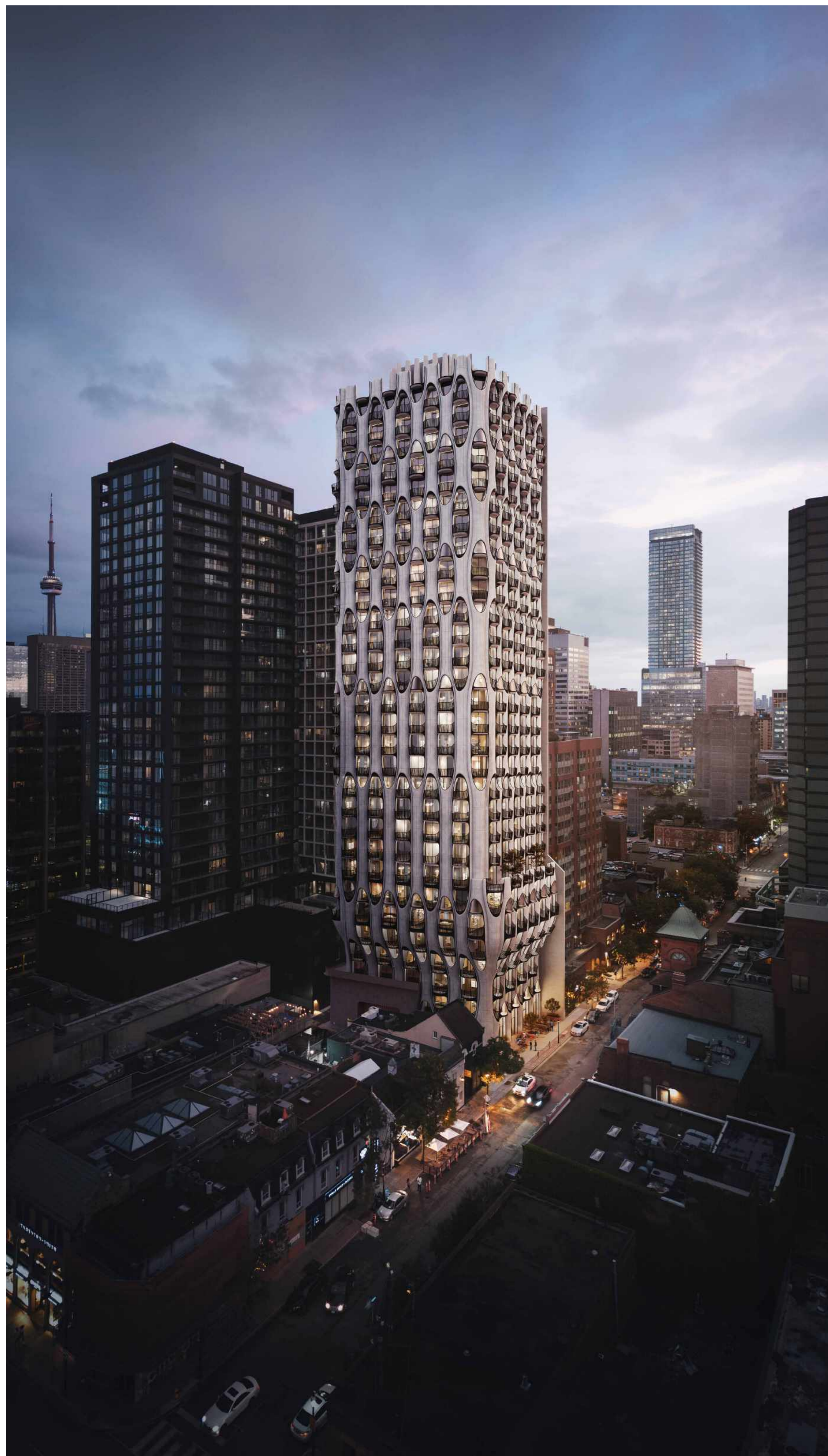
2 Aerial View of Building looking Southwest A4001 1:1
