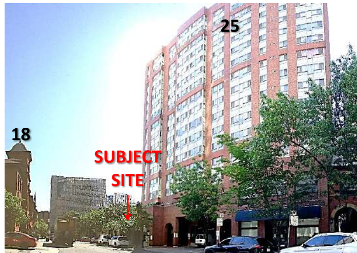
13. View easterly along Elm Street
