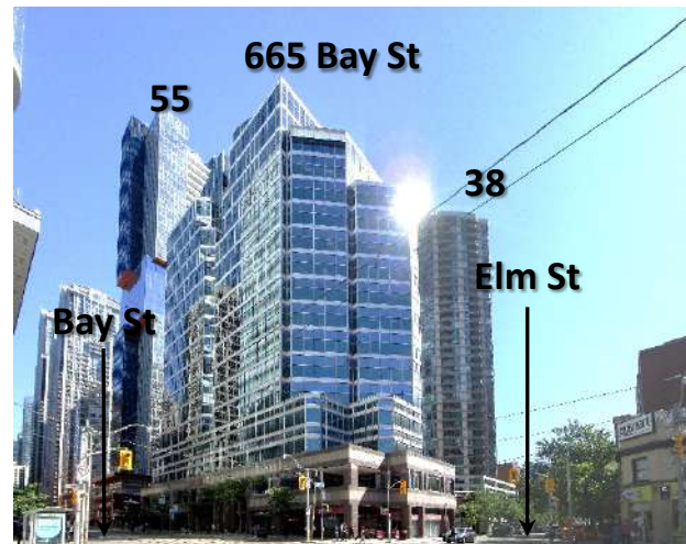
14. View northeasterly from Bay Street and Elm Street intersection
