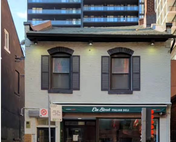
Figure 57: Built up roof system with pebble surface (ERA, 2022).
