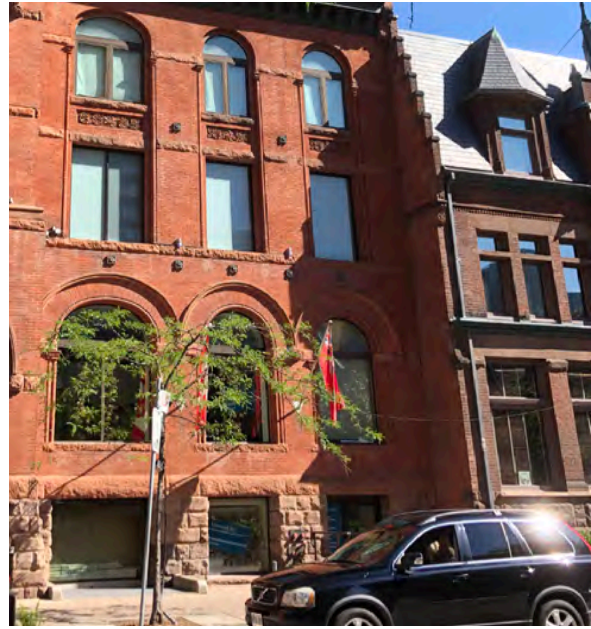
Figure 30: Partial west elevation (ERA, 2022).
