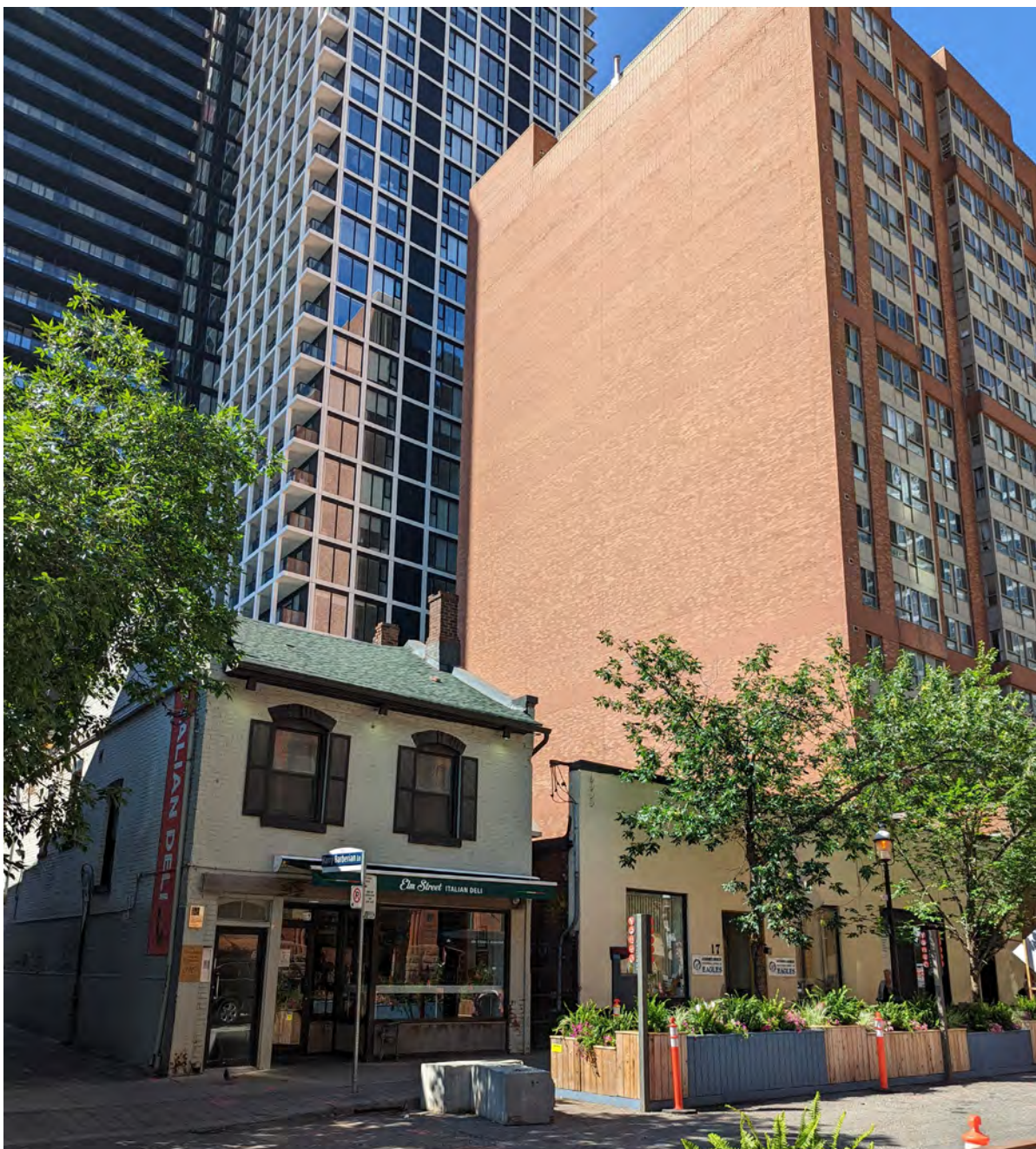
Figure 14: Context photo of the Site looking south from Elm Street (ERA, 2022).
