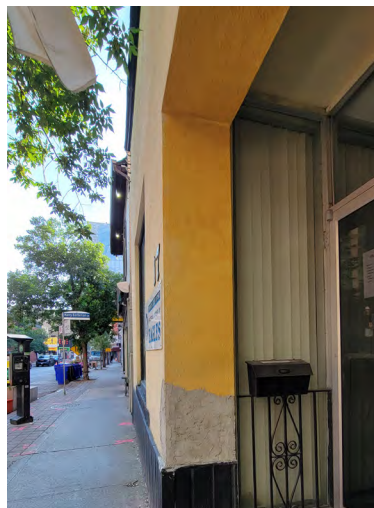
Figure 65: Stucco and cement repair (ERA, 2022).
