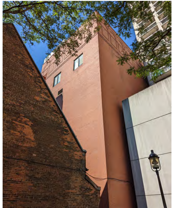
Figure 36: Partial north elevation (ERA, 2022).
