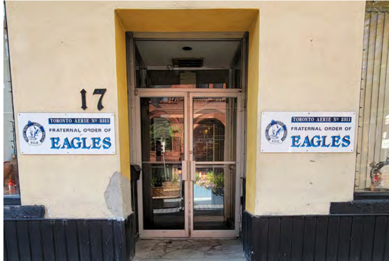
Figure 63: Aluminium doors and vestibule with glazing in fair condition. Cement stucco repairs visible. Stone step is in poor condition (ERA, 2022).
