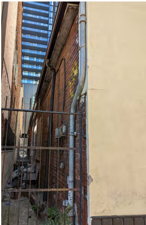
Figure 22: Partial east elevation (ERA, 2022).
