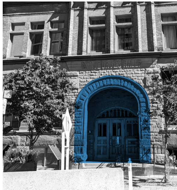
Figure 88: The south facade of 14 Elm Street (ERA, 2022).
