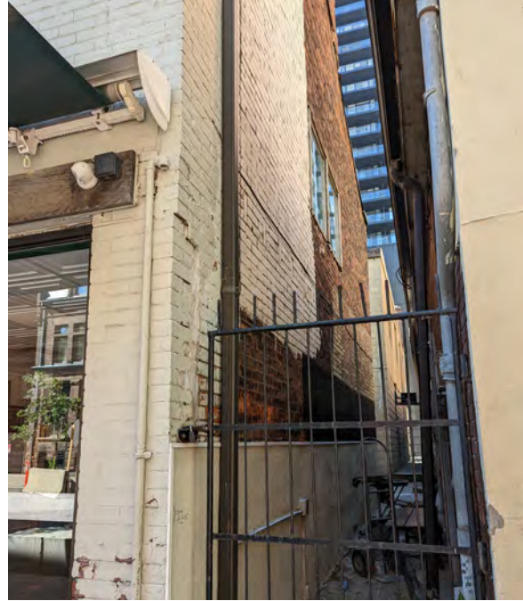
Figure 18: West elevation (ERA, 2022).
