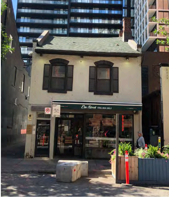
Figure 17: North elevation (ERA, 2022).
