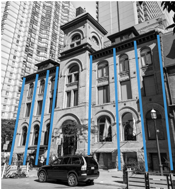
Figure 84: The south facade of 18 Elm Street (ERA, 2022).
